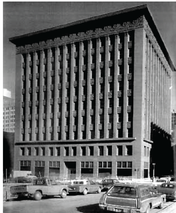
1890-91 Wainwright Building, St. Louis, Louis Sullivan
